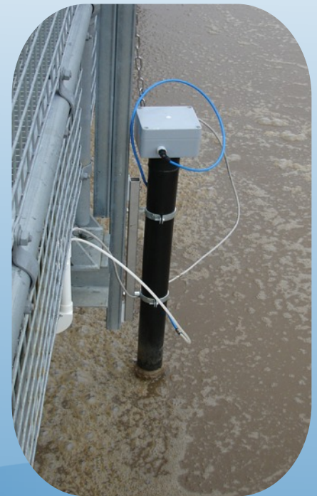
Installation on plug flow aeration unit for DO set point control
