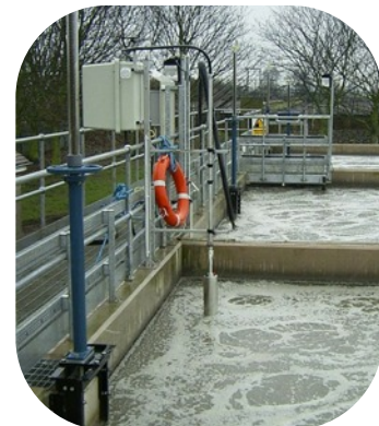
PBS1 in use in final effluent
