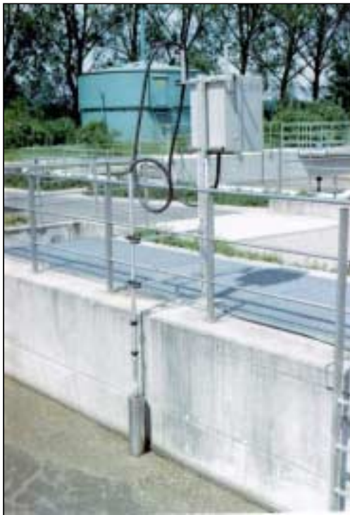
Buoy installed in aeration basin
