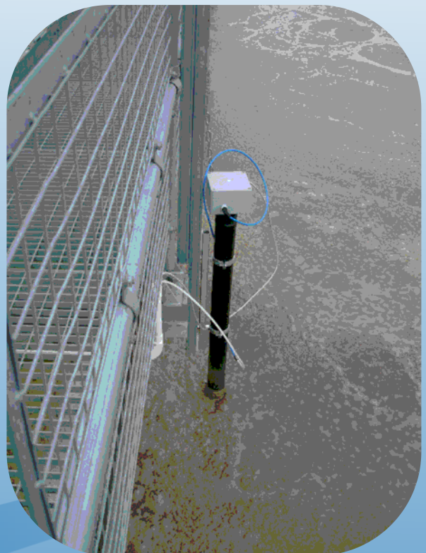
Installation on plug flow aeration unit for DO set point control
