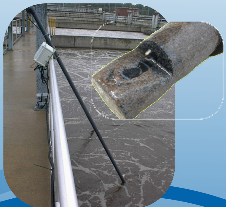
Diffused air Activated Sludge Plant monitoring and control Sensing area is kept clean by air jet
