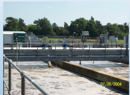
Typical Application: ASP process control
