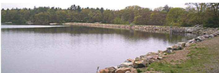
LILY POND HOLDING RESERVOIR AT THE COHASSET WATER TREATMENT PLANT
